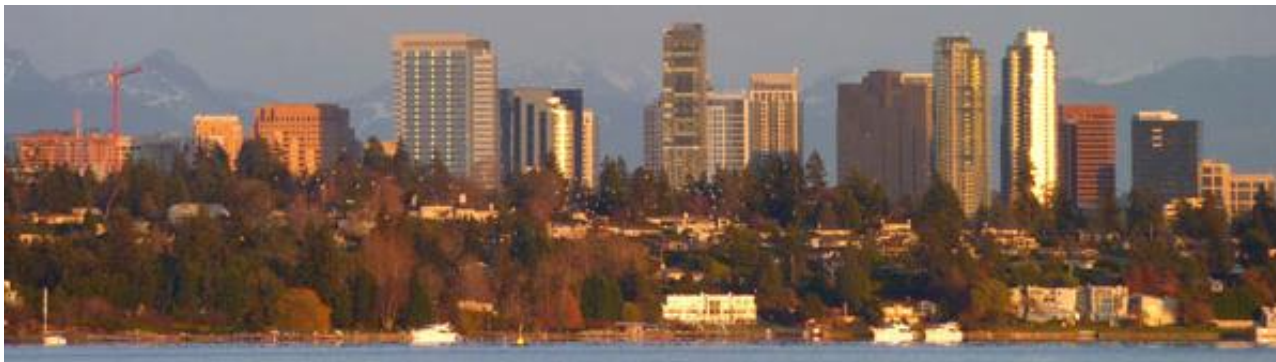
FIGURE 15. Downtown's skyline, when viewed from a distance, lacks much visual interest in terms of rooftop forms.
